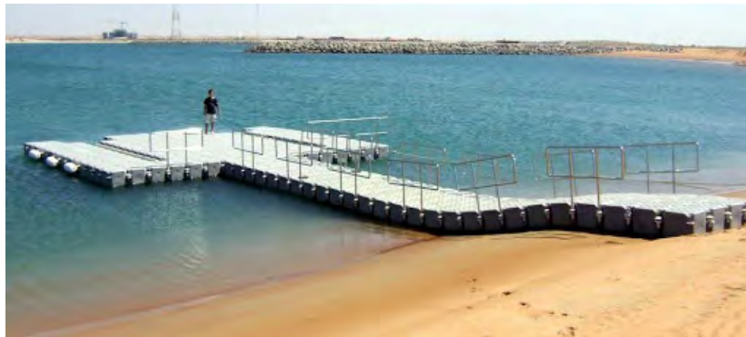
Figure 41. Floating Pontoon Pier (KKCL, n.d.)
