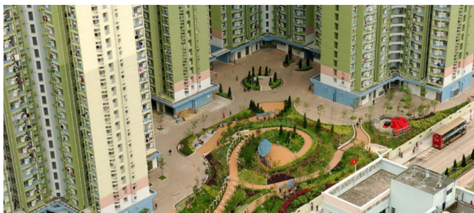
Figure 8-27: Greening Area in Un Chau Estate Source: Hong Kong Housing Authority, 2020
